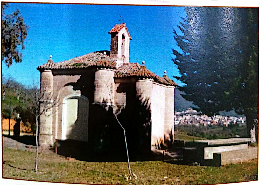
General view of the chapel.
